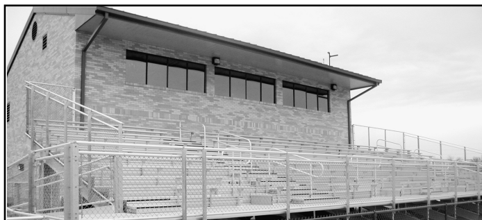
Track & Field Complex
